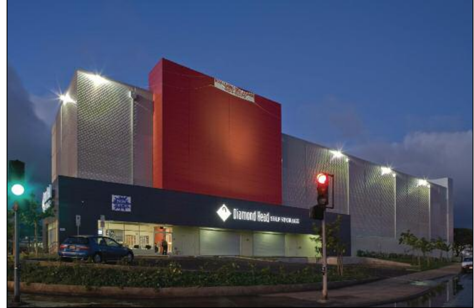
ABOVE: The Diamond Head Self Storage, in Honolulu. In an effort to provide a sustainable design, RIM Architects created a building that uses the footprint of the existing building and 50 percent of the existing walls as well as solar energy panels.
